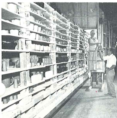
(7) Stacking kiln for firing.
